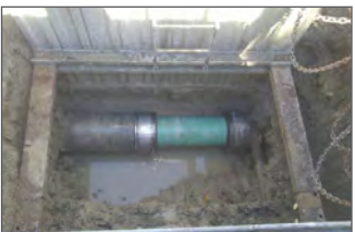
Sewer Line Repair
