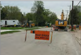
Barkman Avenue Reconstruction
